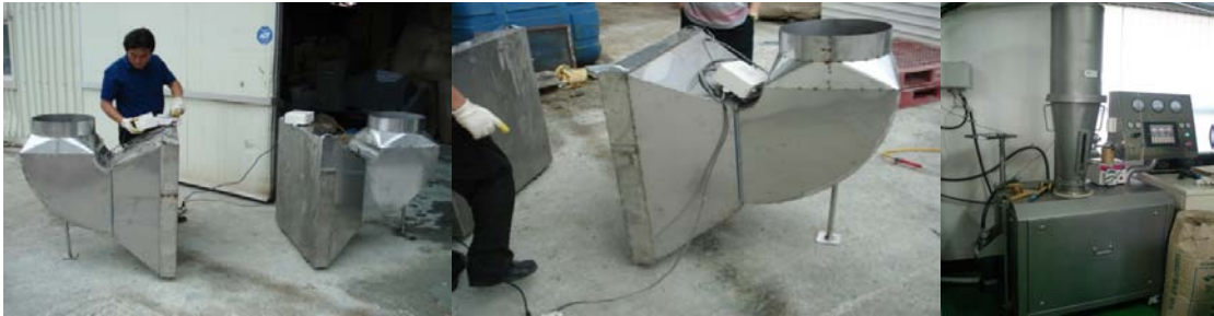
LUMILITE Deodorization Facility
